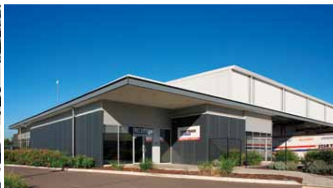
32 SARGENTS ROAD, MINCHINBURY, NSW
