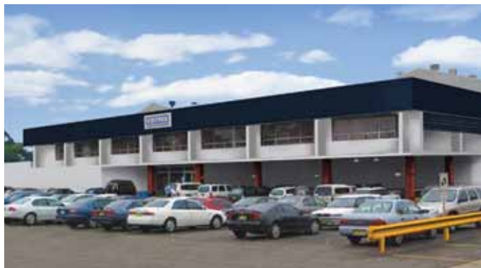
64 BILOELA STREET, VILLAWOOD, NSW
