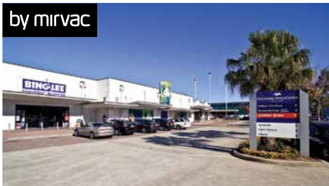
BLACKTOWN MEGACENTRE, BLACKTOWN, NSW
