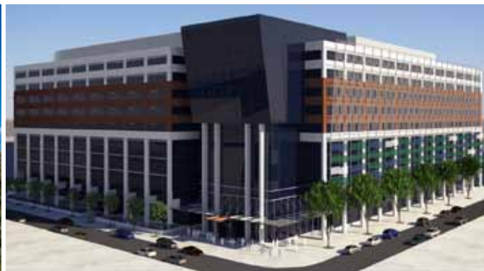
SIRIUS BUILDING 23 FURZER STREET, PHILIP, ACT
