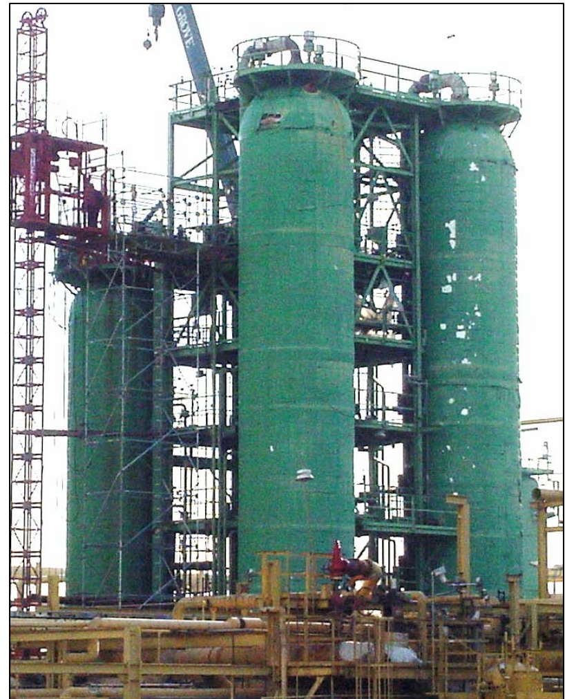
Hydrocracker Reactors
