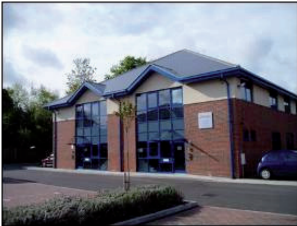
Global Technical Centre (GTC) – Horsham UK
