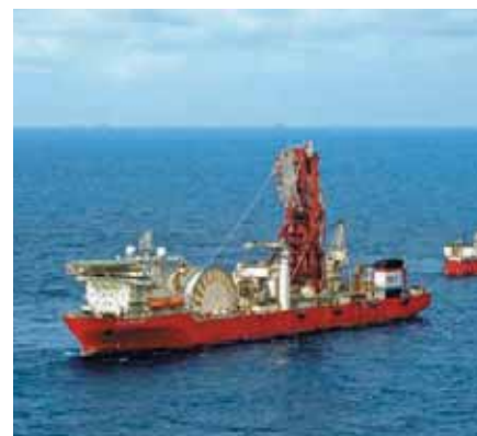
Technip's 677-foot construction vessel, Deep Blue, the largest ultra-deepwater reeled subsea construction vessel in the industry, operating in 6,700 feet of water installing the flowline connecting Mariner Energy's Bass Lite project to Williams' Devils Tower floating production facility.
