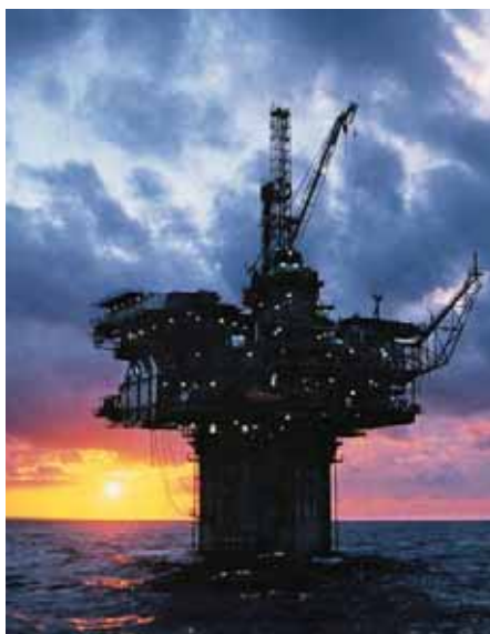
Anadarko's Nansen spar, located in 3,680 feet of water, hosting Mariner Energy's production from the neighboring Anadarko-operated Northwest Nansen deepwater field in which Mariner owns working interests ranging from 33% to 50%.
