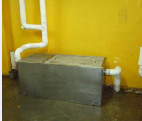
New Grease Trap for Loading Bay 2
