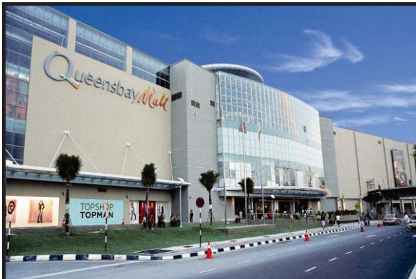
Queensbay Mall 2 , Penang
