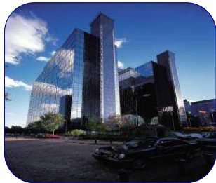
Exchange Tower, London E14
