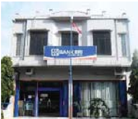
Sub-Branch Office Tugumulyo, Ogan Komeringlilir, South Sumatra
