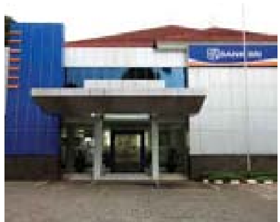
Branch Office Cut Mutia, Jakarta
