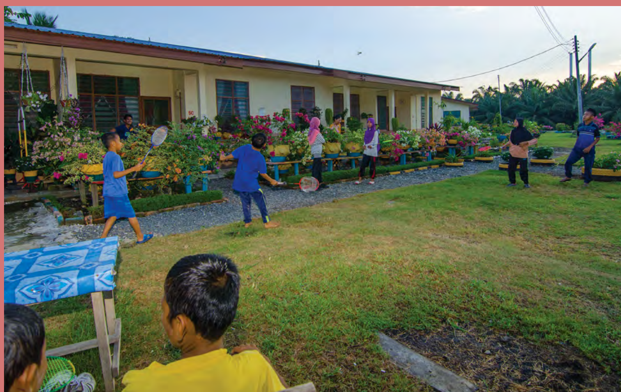
Plantation workers' housing complex
