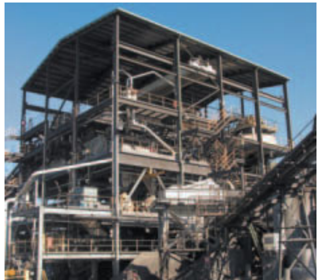
THE COPPABELLA MINE COAL HANDLING AND PREPARATION PLANT
