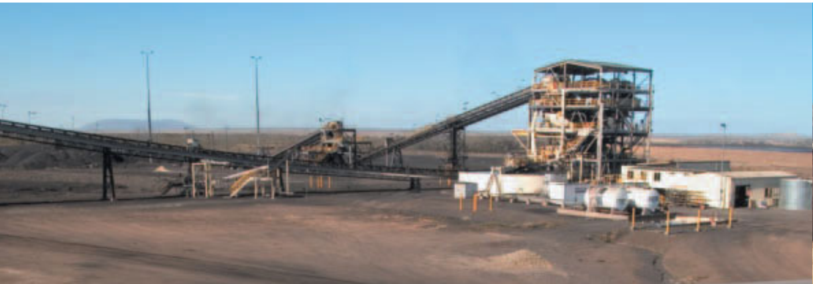
MOORVALE MINE COAL HANDLING AND PERPARATION PLANT
