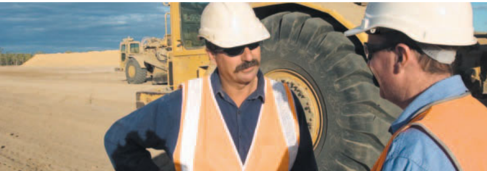
SCOTT GOLDING, ENVIRONMENTAL COORDINATOR AND GUS WINDSOR, SCRAPER OPERATOR, DISCUSSING TOPSOIL REMOVAL PRIOR TO MINING OPERATIONS
