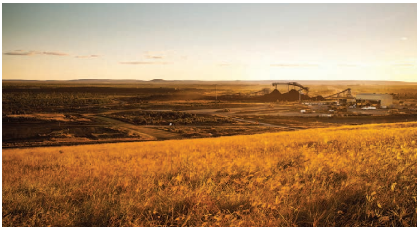
Dusk at Moorvale Mine – overlooking the CHPP and maintenance workshop with rehabilitated pastures in the foreground.
