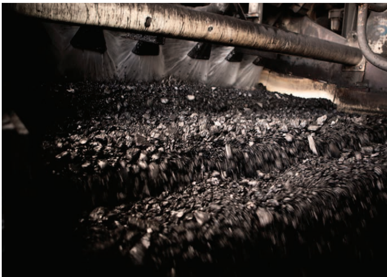
Action shot from inside Coppabella's CHPP - coal being processed through the plant's feed desliming screen.
