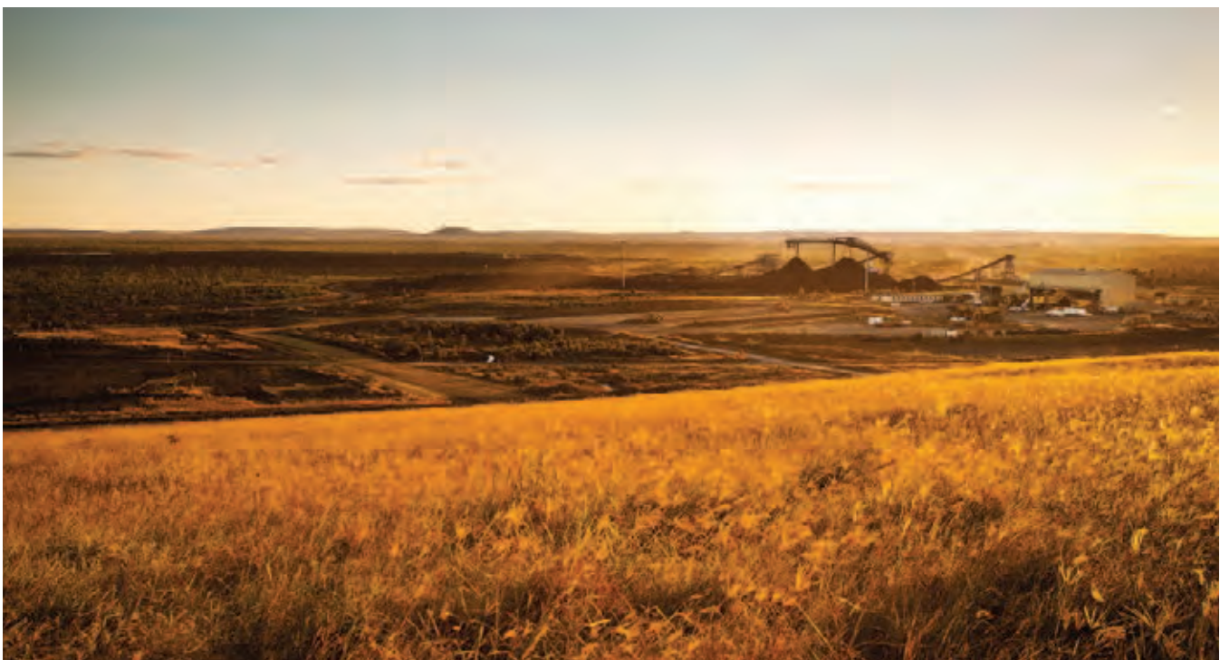
Dusk at Moorvale Mine – overlooking the CHPP and maintenance workshop with rehabilitated pastures in the foreground.
