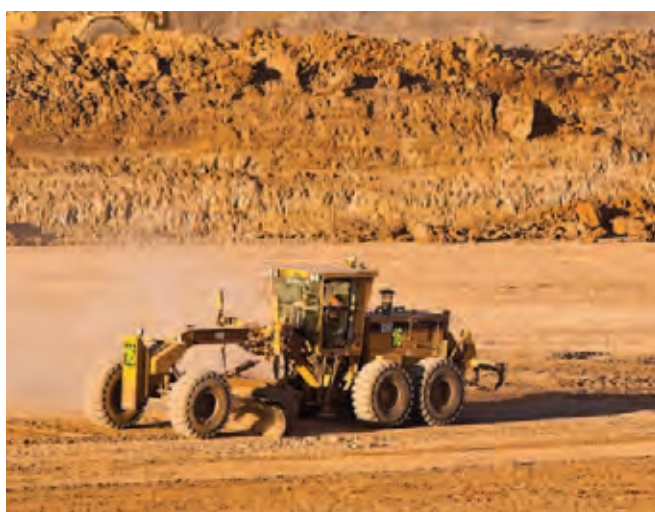
Grading roads at Moorvale Mine – maintaining road conditions is crucial to improving safety, productivity and tyre life. The focus on road maintenance was heightened during recent wet weather.
