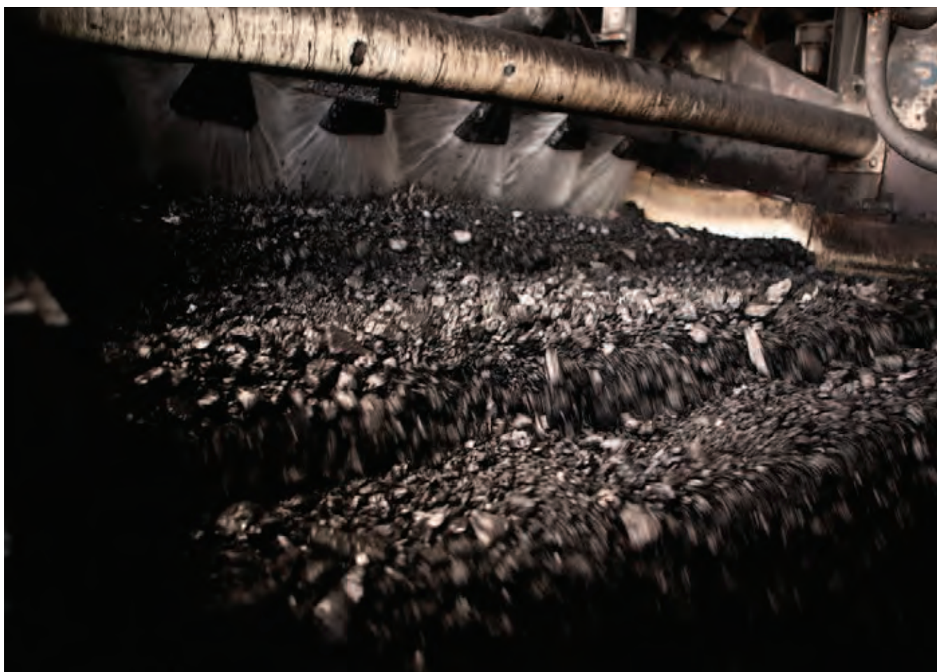
Action shot from inside Coppabella's CHPP - coal being processed through the plant's feed desliming screen.
