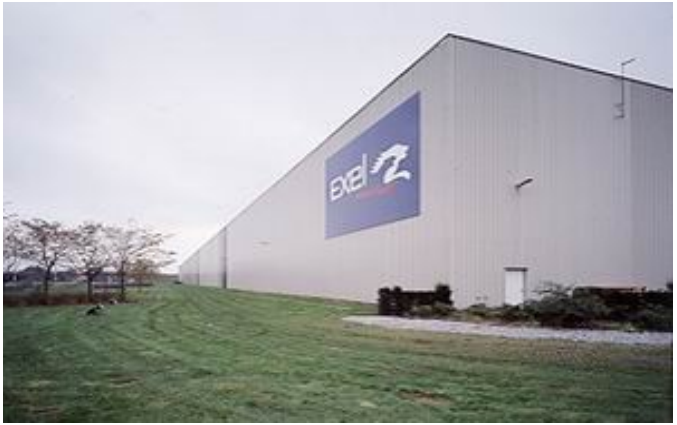
Location: Wommelgem, Belgium (24,099 m 2 )
