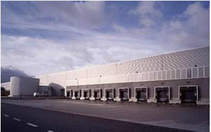
Location: Tilberg, the Netherlands (80,874 m 2 )
