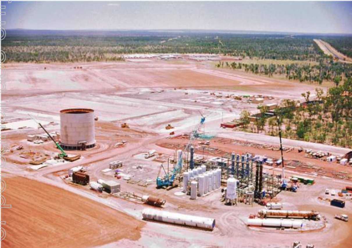
Re-construction of the ammonia plant and new ammonia tank, with power plant, evaporation ponds and camp site in background (late 2007)
