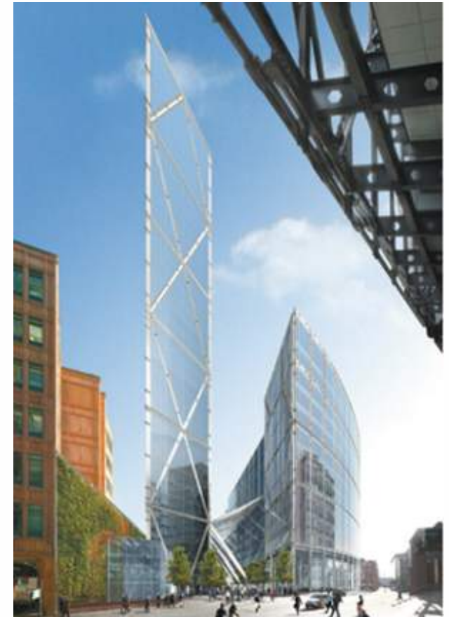
201 Bishopsgate and Broadgate Tower
