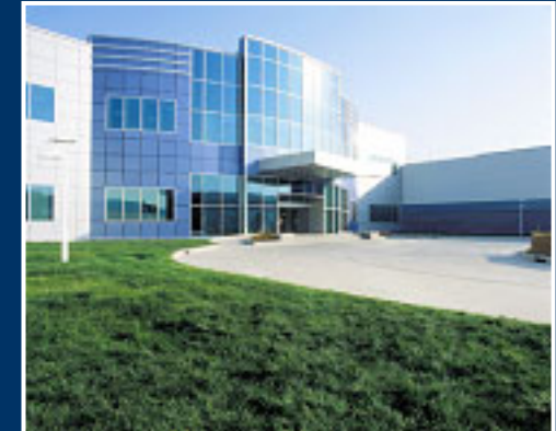
CTS New Manufacturing Facility, Tianjin
