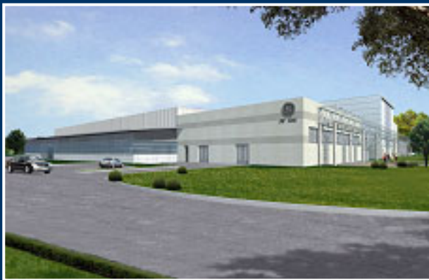
GE Betz New Facility, Wuxi
