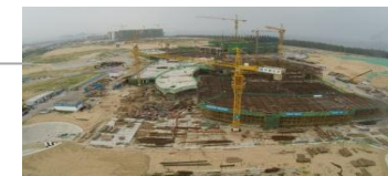
Construction progress image for Atlantis, Hainan, Sanya
