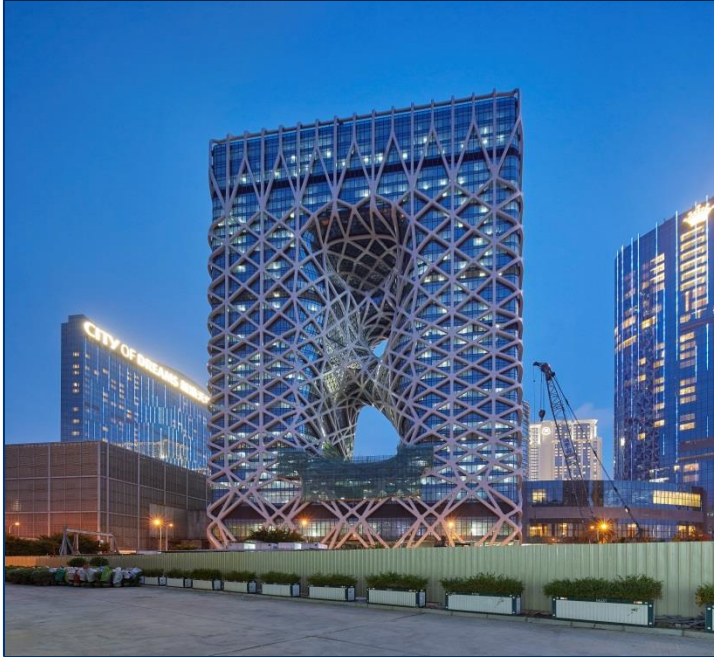
Image: Latest Construction Update
