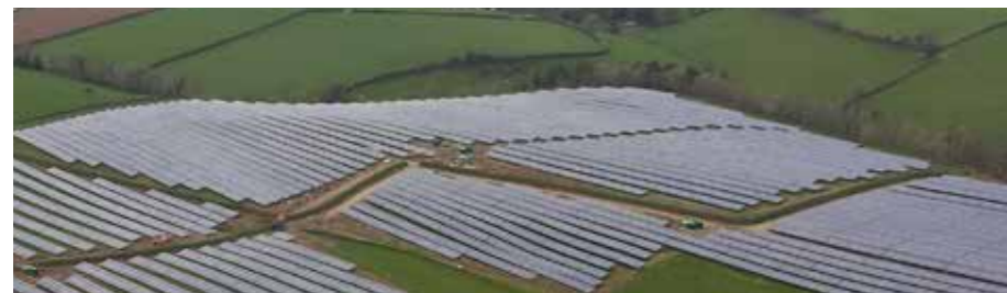
⬆️ Trehawke project, UK 10.6 MW Completion date: 2014/03
