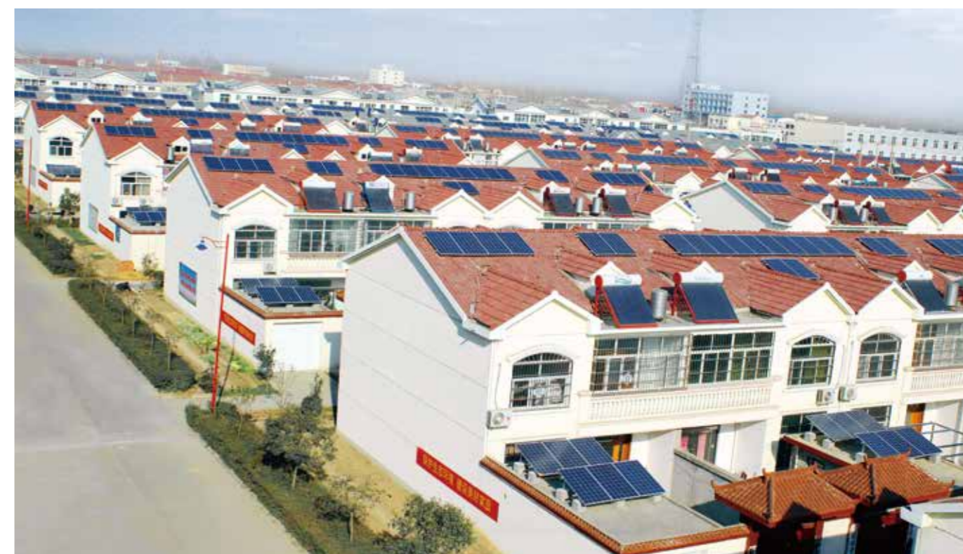
381.2 KW DG Project, Lianyungang, Jiangsu Province, China
