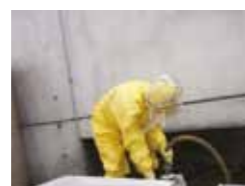
Tracing leak source
