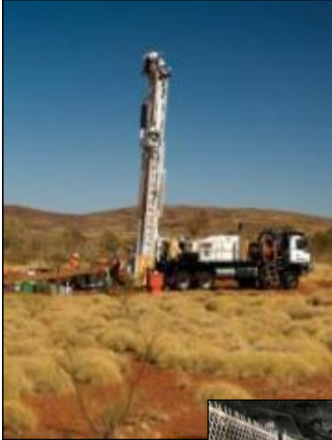
Diamond Core Drilling (Surface & Underground)
