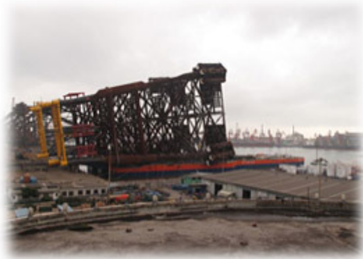
Jacket on launch barge
