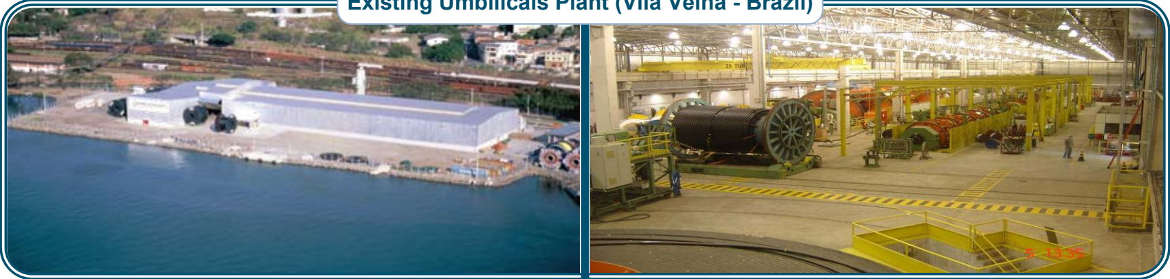
Existing Umbilicals Plant (Vila Velha - Brazil)
