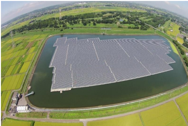
One of the world's largest floating mega solar projects was completed in Japan by one of our partners. Project size: 7.5 MW Connected on October 26, 2015 Location: Saitama Prefecture, Kawajima City Modules: PANDA 275w x 27,456 Modules
