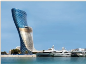
Hyatt at Capital Gate, Abu Dhabi 189 Rooms 4Q 2011
