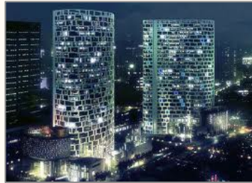
Andaz Shanghai 307 Rooms 4Q 2011
