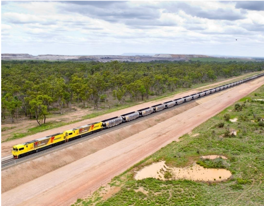
First coal train to cross the Northern Link on 19 December 2011
