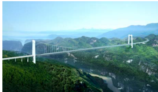
Lishui Grand Bridge Hunan Province, China
