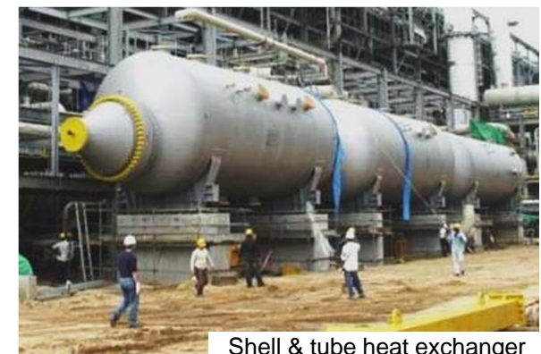
Shell & tube heat exchanger
