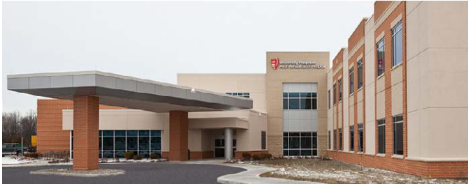
UH Rehabilitation Hospital – Avon, OH 54,800-square-foot rehabilitation hospital for University Hospitals and Kindred Healthcare
