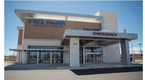
SCL Emerus Littleton – Littleton, CO 37,000-square-foot, 100% leased community hospital
