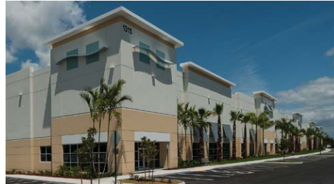
Turnpike Crossing 1315 – West Palm Beach, FL 124,500-square-foot speculative warehouse delivered Q2; 61% leased
