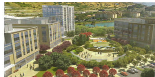
The Cove at Oyster Point Life Science Development (rendering) South San Francisco, CA
