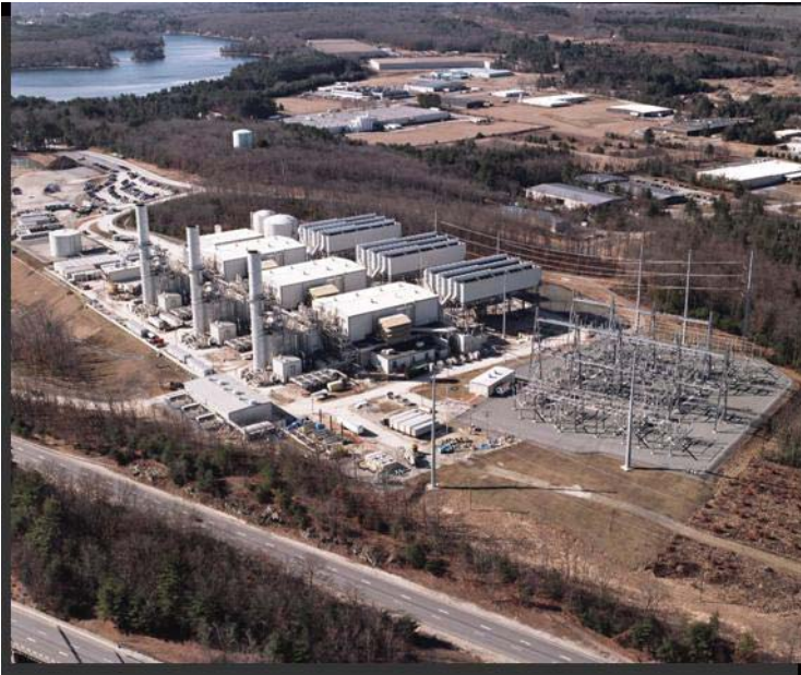
Lake Road Power Plant Dayville, Connecticut 750 MW
