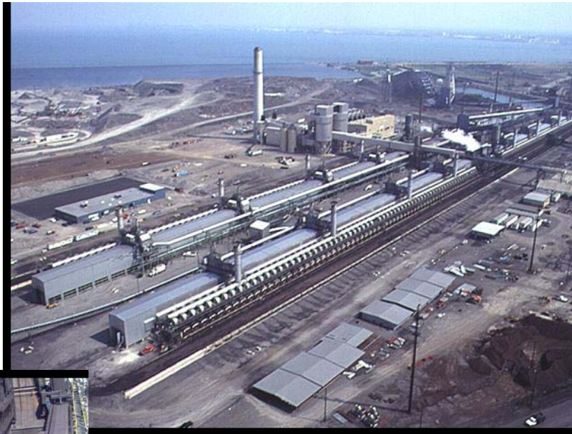
Indiana Harbor Coke Battery East Chicago, Indiana
