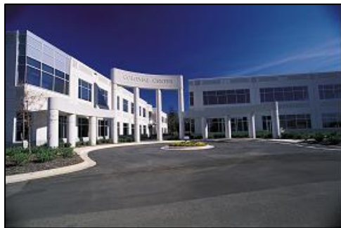
Colonial Center at Research Park Huntsville, Alabama
