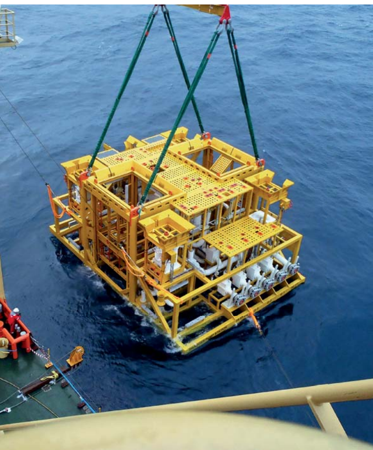
View of a multiphase subsea pump installation in the Shell Draugen field in the North Sea. The system integration of Framo pumps represented the world's first commercial subsea multiphase pump installation.
