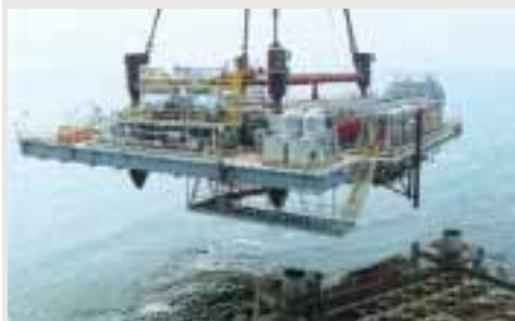
Installation of the offshore platform deck on the Sanha Bomboco project
