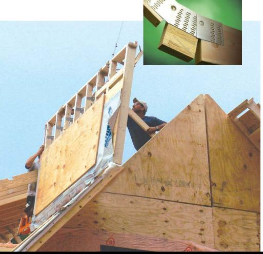
Universal's patented Double Hinged Plate allows peak caps to be factory installed and unfolded at the building site. In addition to offering more design options for homes constructed with factory built components, the DHP $^{\text{TM}}$  saves labor and expense. More and more builders want this new Universal technology.
