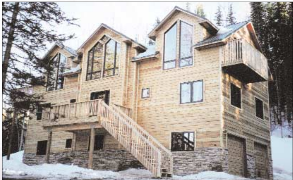
All American KanBuild designed and built this custom modular home in Colorado. With three floors and nearly 4,000-sq. ft of living space, this spacious home has vaulted ceilings, a U-shaped staircase, two fireplaces, four bedrooms, sun deck and balcony.
