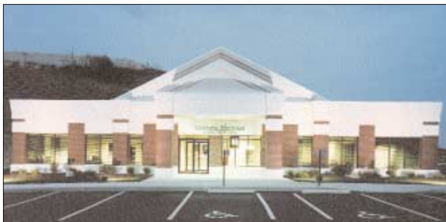
Miller Building Systems specializes in commercial structures such as telecommunications buildings, schools, multi-story office buildings, medical buildings and banks. Miller and its customer, New Ground Resources, Inc, constructed this bank building.
