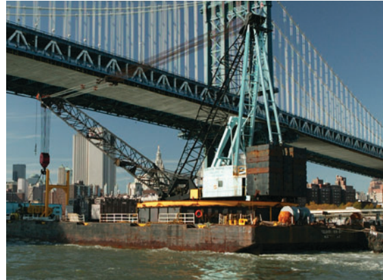
The transformers for 7 World Trade Center, which traveled by barge down the East River, will provide reliable electric power to Lower Manhattan now and in the future and are part of a multi-year, $430 million investment for Con Edison.
