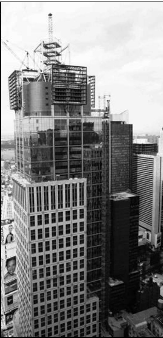
The New York City real estate market is booming, making building cranes a frequent skyline feature, as seen here in Times Square
