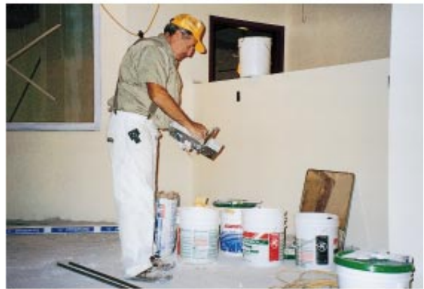
A recently built community center prior to its Grand Opening (top). Renovations which enhance the quality of life for residents also receive premium rents and improve occupancy rates (bottom).
