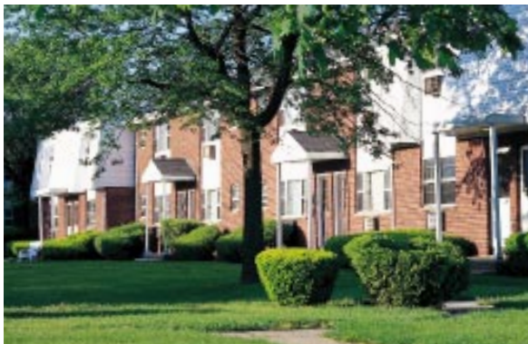
Pleasantview Apartments, 1,142-units, in Piscataway, NJ
