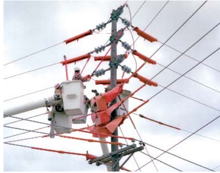
Chance insulated conductor covers help protect line personnel from accidental contact with energized power lines.
