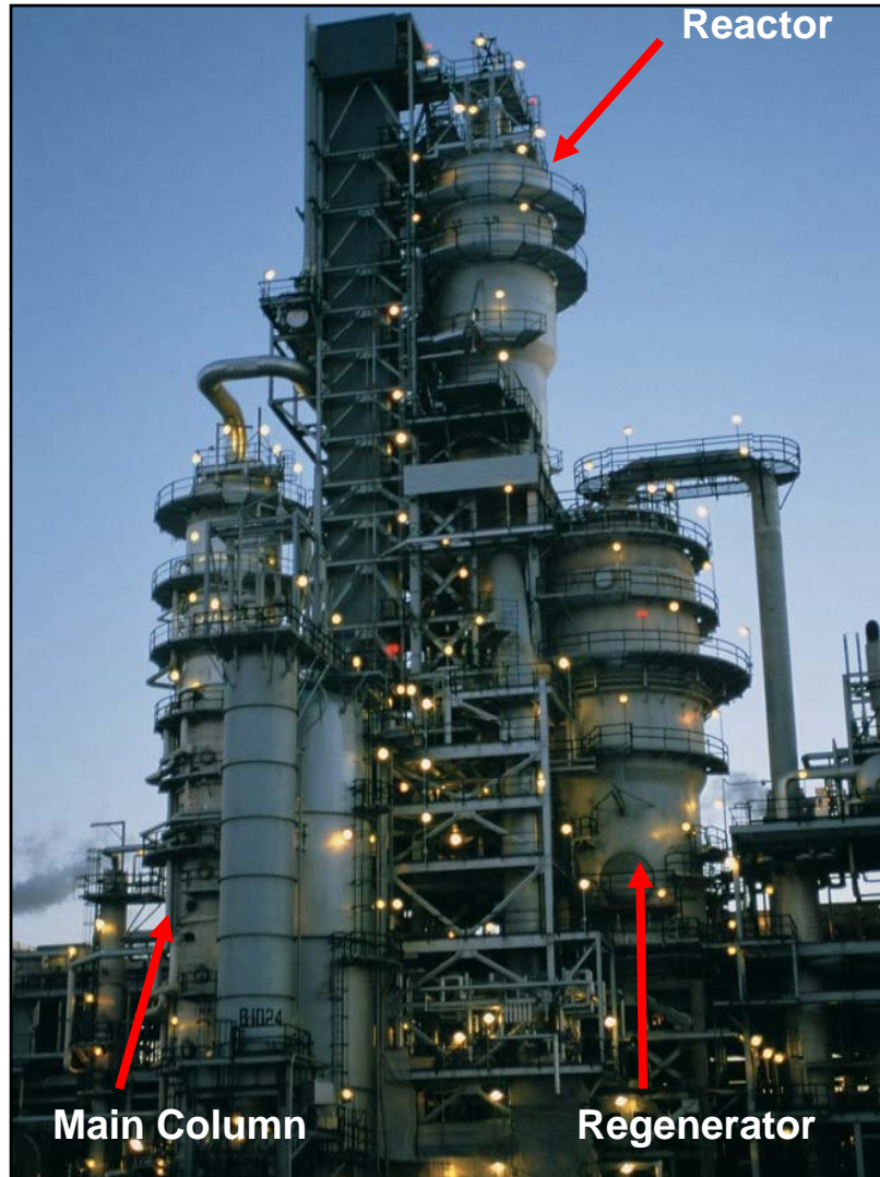
Fluidized Catalytic Cracker
