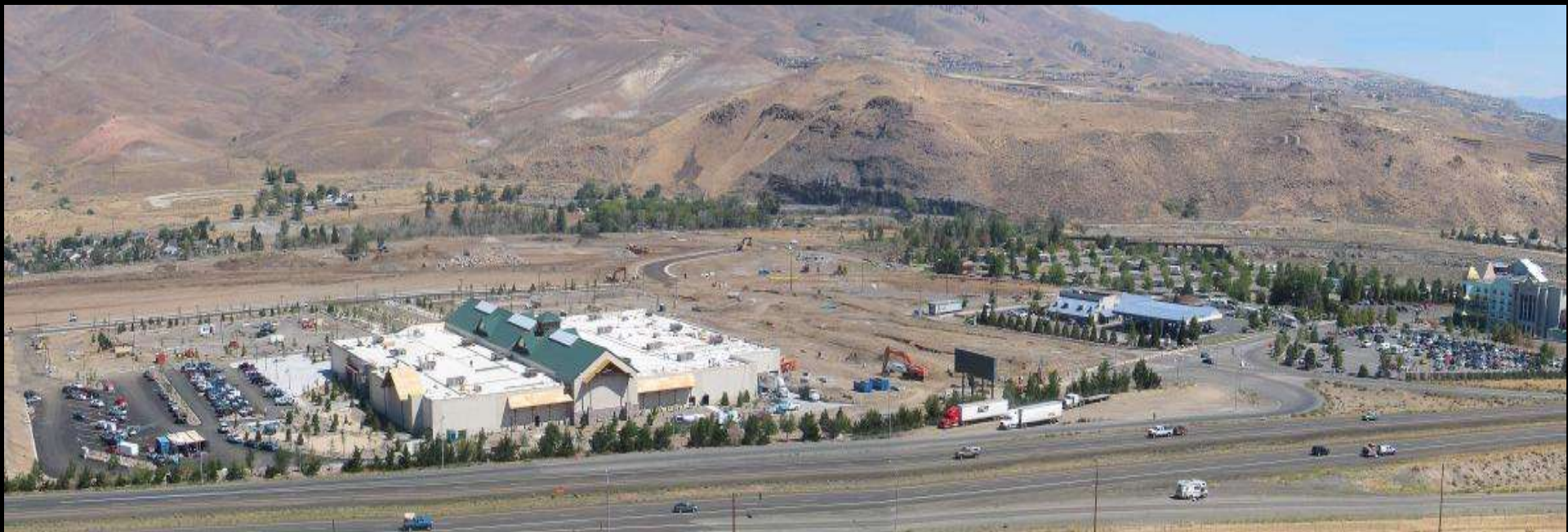
Boomtown Reno Construction of Adjacent Cabela's Retail Store
