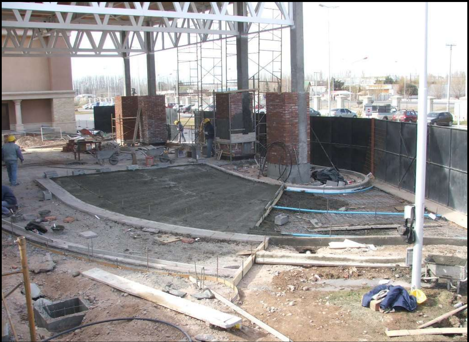
Casino Magic Argentina Hotel Construction
