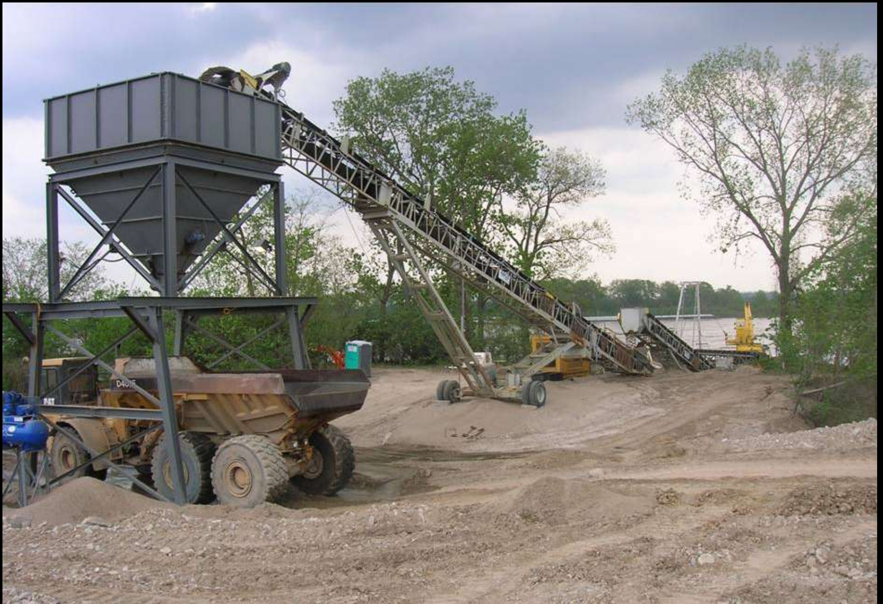
River City: Project Site
