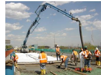
Passaic River Bridge Newark, NJ
