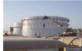
Water Tank Construction LSA Anaconda Iraq
