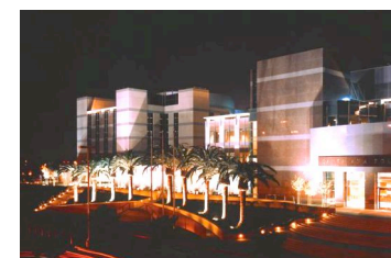
Police Administration and Jail Santa Ana, CA
