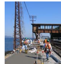
Metro North Commuter Rail Line Rehab Project New York
