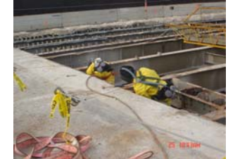
Bridge Work Cherry Hill Construction
