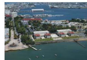
Personnel Housing U.S. Coast Guard Puerto Rico
