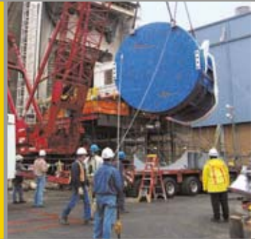
Above: The old vessel head is removed.
