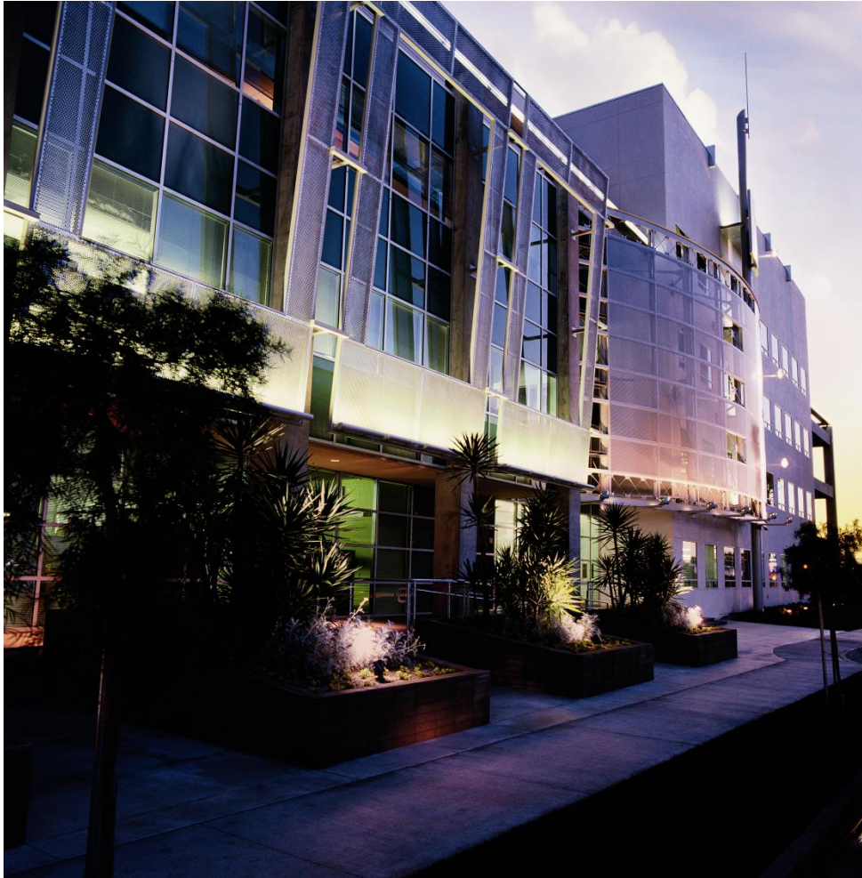
West Side Media Center, Los Angeles
