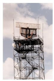
Under contract with the U.S. Federal Aviation Administration (FAA), Northrop Grumman delivered 134 ASR-9 airport surveillance radars. The company's newest solid-state primary surveillance radar system is the ASR-12, which evolved from the ASR-9 and is now operational in Mexico, Peru and El Salvador. Nine additional systems are scheduled for delivery to three other countries.
