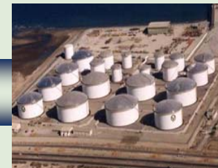
Tank Farm and Plant Construction
